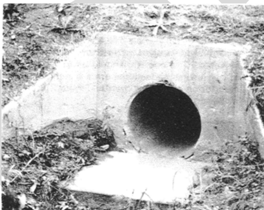
Figure 7.29 (a): Headwall and Wingwall Inlet
