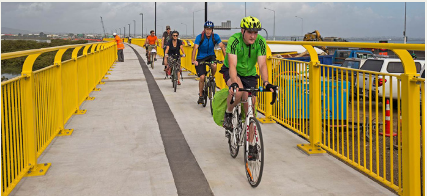
SH16 Causeway Cycleway
