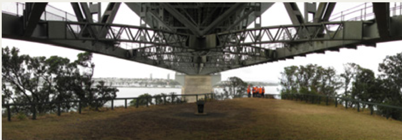
Te Onewa Point, under the Auckland Harbour Bridge
