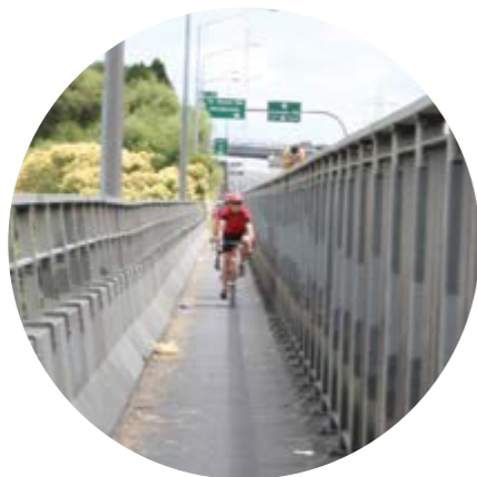
Auckland's Western Cycleway: Inadequate facilities for pedestrians and cyclists on bridge.
