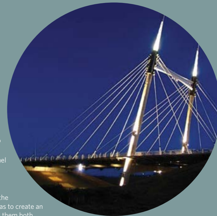
Feature lighting: Ormiston Road Bridge, Auckland Lighting needs to be thought about in the early phases of a project, to ensure that it is captured in the business case and funded.
