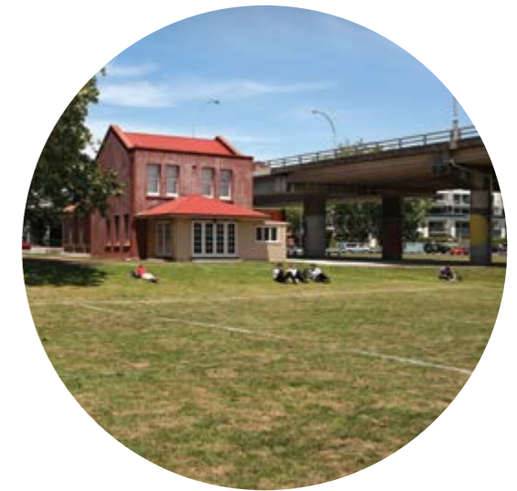
Campbell Kindergarten: historic building restoration for adaptive reuse, as part of the Victoria Park Tunnel project, Auckland. Photographer: Simon Devitt
