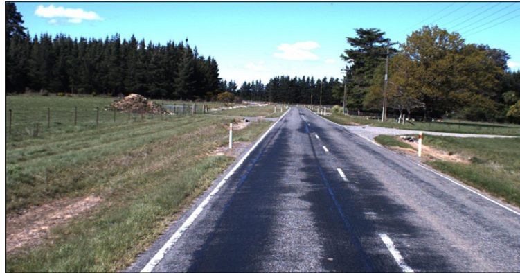
Figure 6: Example of a flushed chipseal surface
