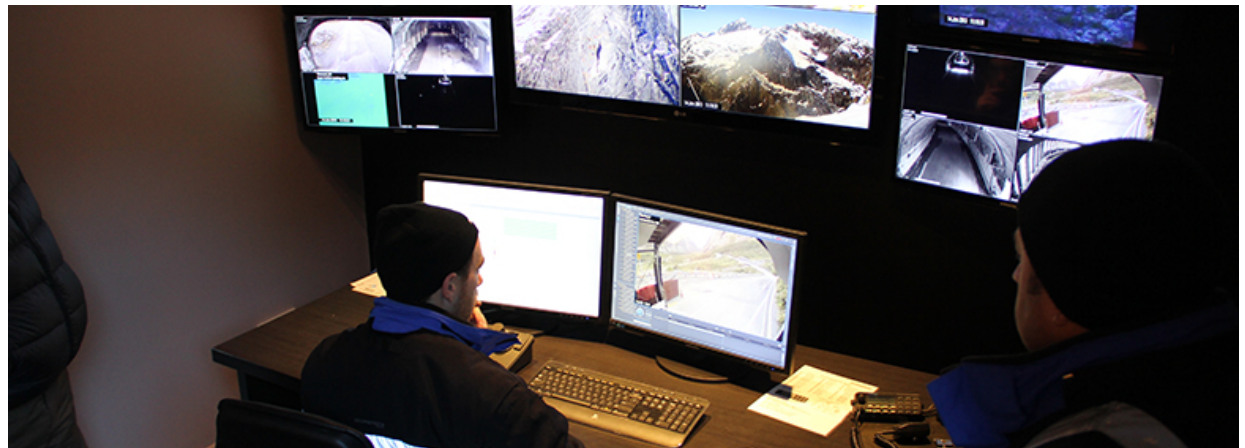
High-tech camera's, Homer Tunnel on State highway 94 to Milford Sound
