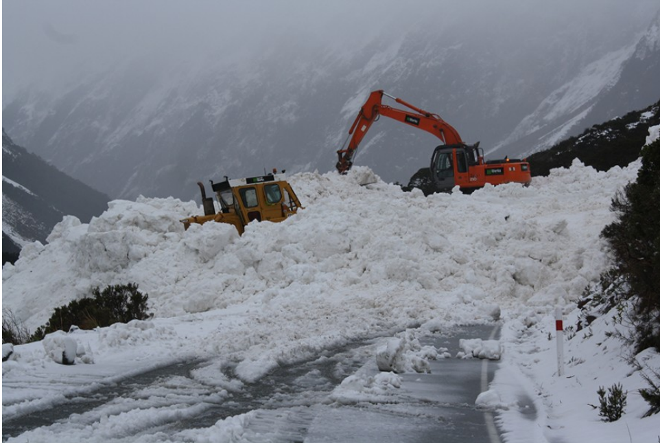
A Digger and dozer clearing snow near the Homer Tunnel
