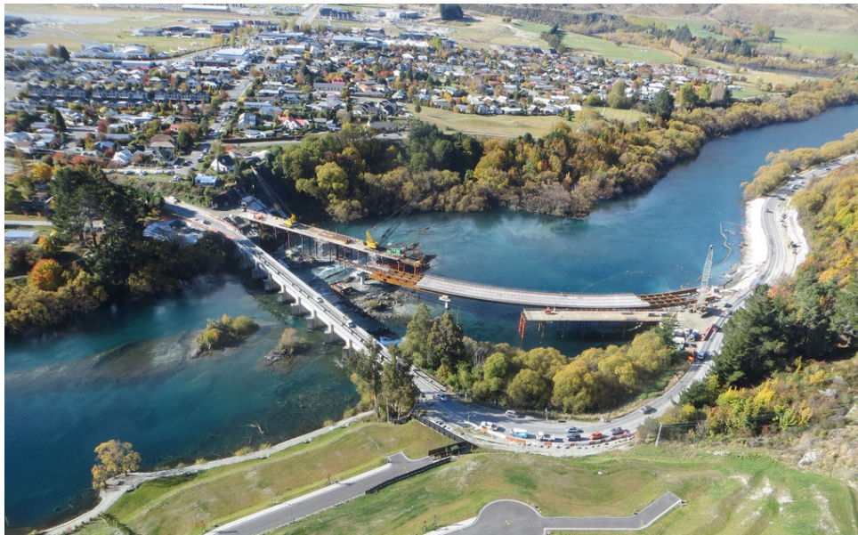
Construction of the new Kawarau Falls bridge is well underway.
