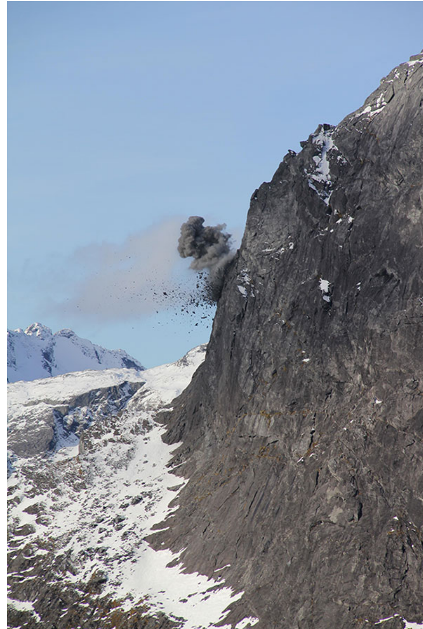
Milford Road proactive rockfall management
