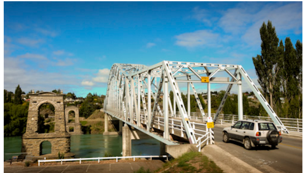
SH8 Alexandra bridge
