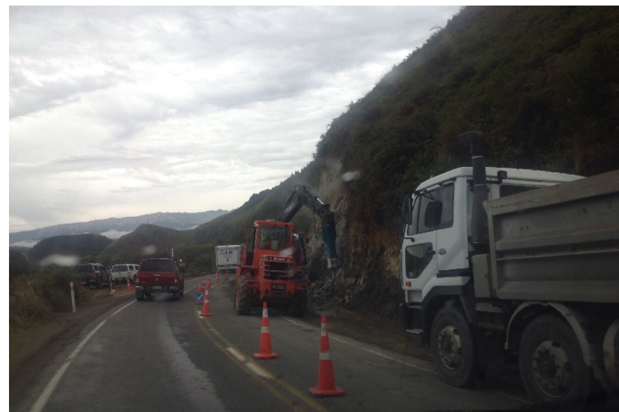
SH63 narrow work site
