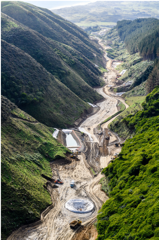
Transmission Gully July 2017
