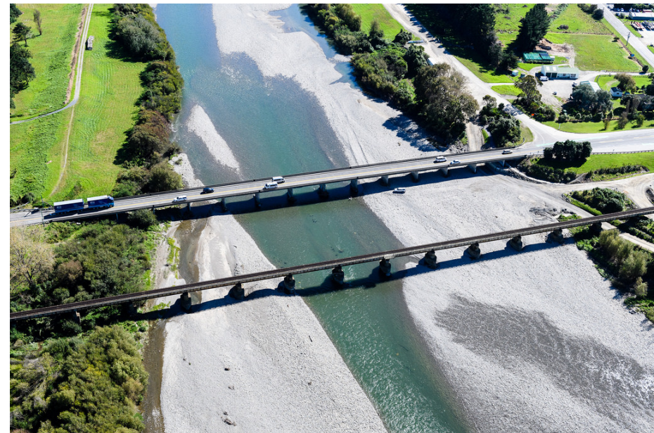
Peka Peka to Otaki expressway
