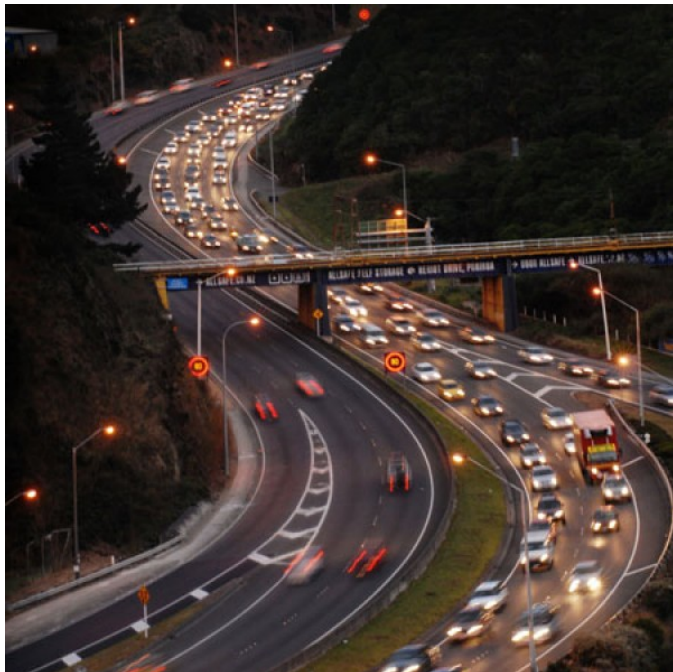
SH1 between Johnsonville and the Terrace Tunnel in Wellington is NZ's first 'smart motorway'
