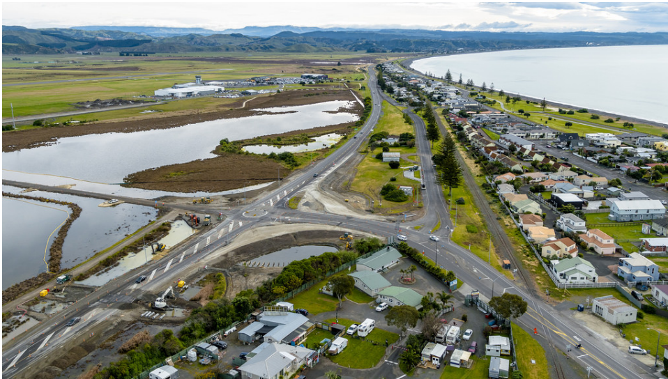
SH2 Watchman Rd intersection, with Napier Airport at left in the distance
