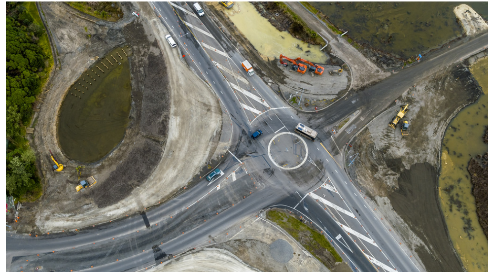
SH2 Watchman Rd intersection aerial view
