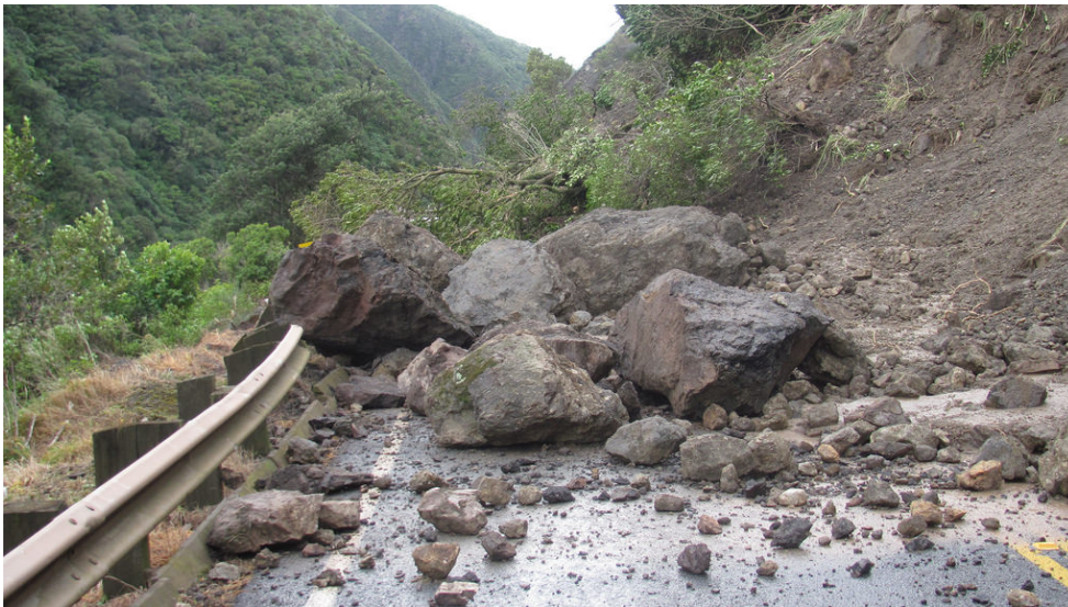
Debris from slip that occurred in the Manawātū Gorge on 23 July 2017
