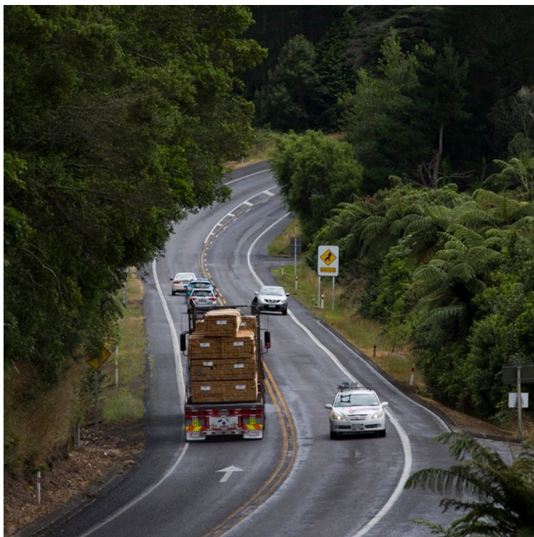
Roadside safety improvements are proposed from the outskirts of Rotorua near Te Ngae, along SH33 to Paengaroa
