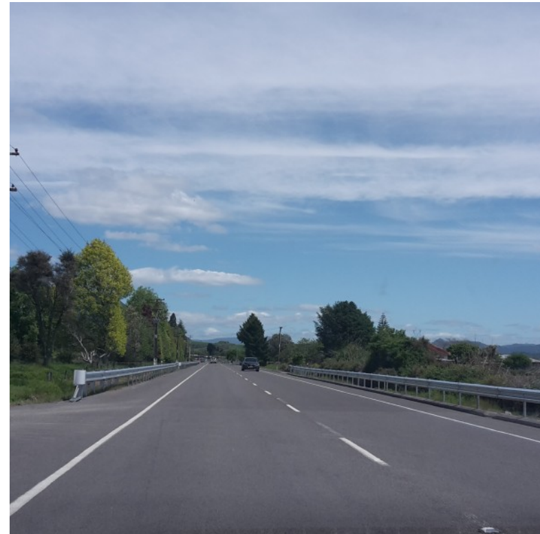
SH30 Te Teko to Awakeri side barriers have been installed in locations where there are roadside hazards and a wide centreline along some of the route to reduce the risk of head-on crashes
