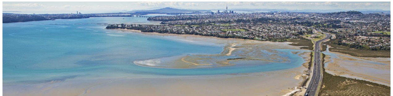
SH16 Causeway upgrade
