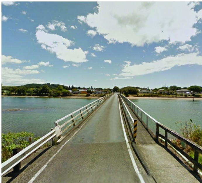
The Taipa bridge is a critical asset which is programmed for improvements to enhance access for pedestrians and cyclists
