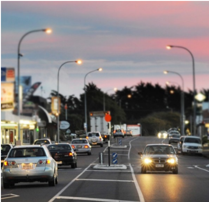
Growth in the region has necessitated improvements to the network at Waipapa to improve safety and facilitate growth
